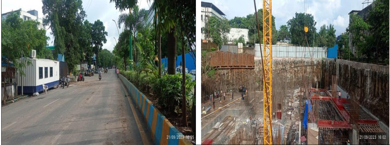
Excavation started on site
